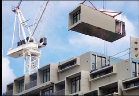
PPVC & PBU Precast
