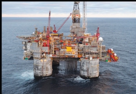
Insulation of Pipeline in Oilfield
