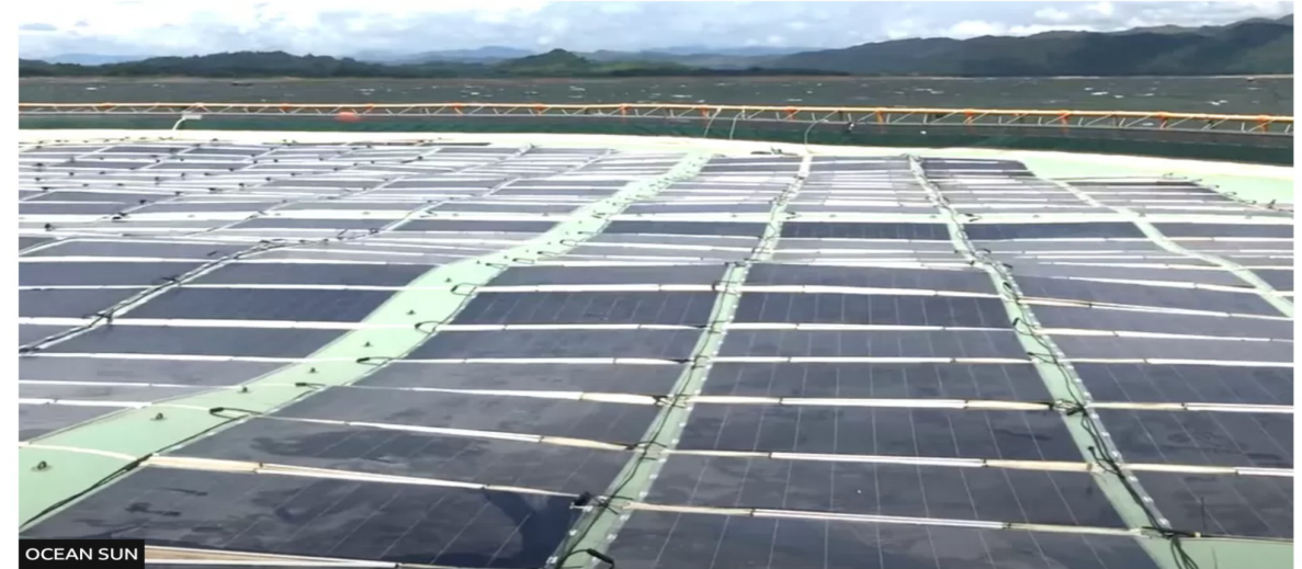
OCEAN SUN The base of the Ocean Solar plant flexes as waves move underneath it
