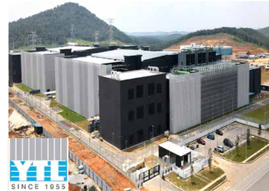
Kulai Green - Data Center, Johor
