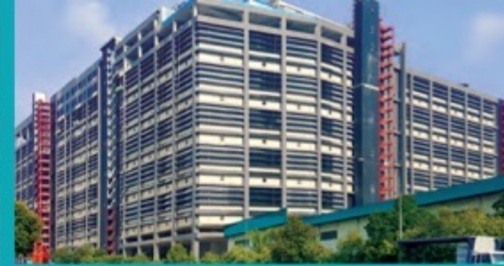
6 Storey Warehouse at 47 Jin Buroh
