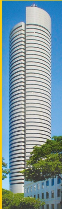
AXA Tower at 8 Shenton Way
