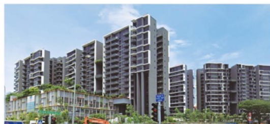
Grandeur Park Residences Condominium
