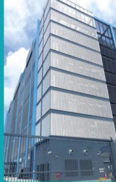
Data Center at Loyang Drive
